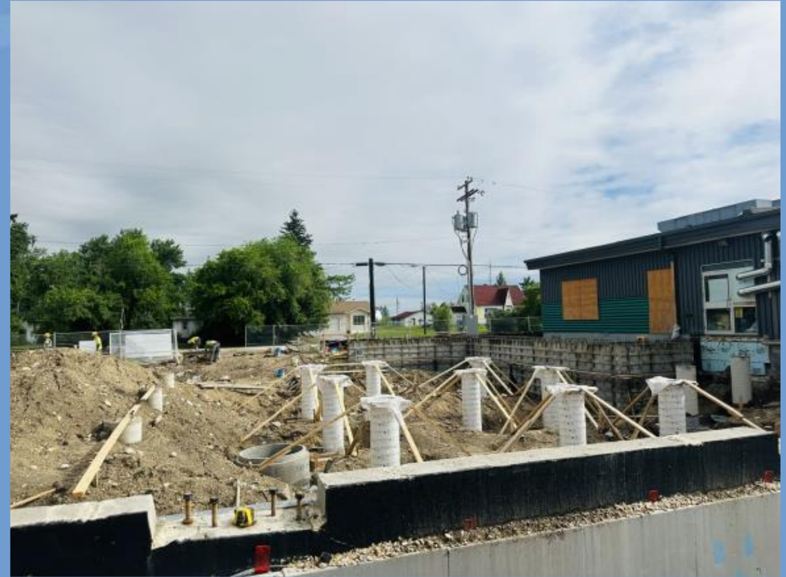
Northeast foundation wall and centre piers
