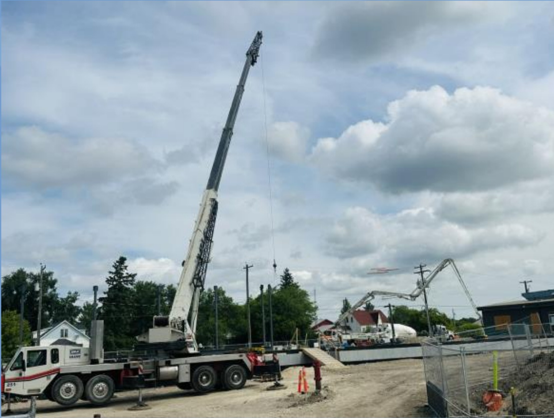
Steel unloading and concrete pouring
